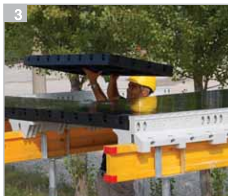
Colocar o painel GEOPANEL® 120
